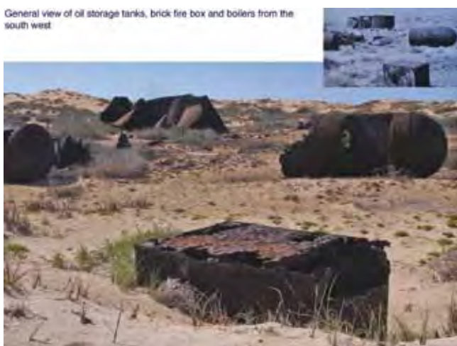
Figure 15. General view of storage tanks, brick fire-box and boilers from the south-west (Colin Cockram).
