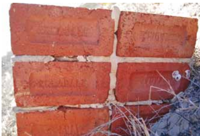
Figure 43. Red clay bricks marked 'ARMADALE' in the frogs (Myra Stanbury).
