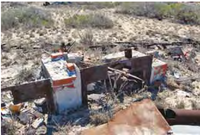
Figure 42. Remains of the Metters stove in the former kitchen and mess facility (Myra Stanbury).
