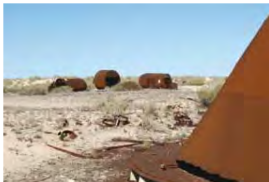
Figure 51. Wall of oil storage tank separated from the base (Myra Stanbury).
