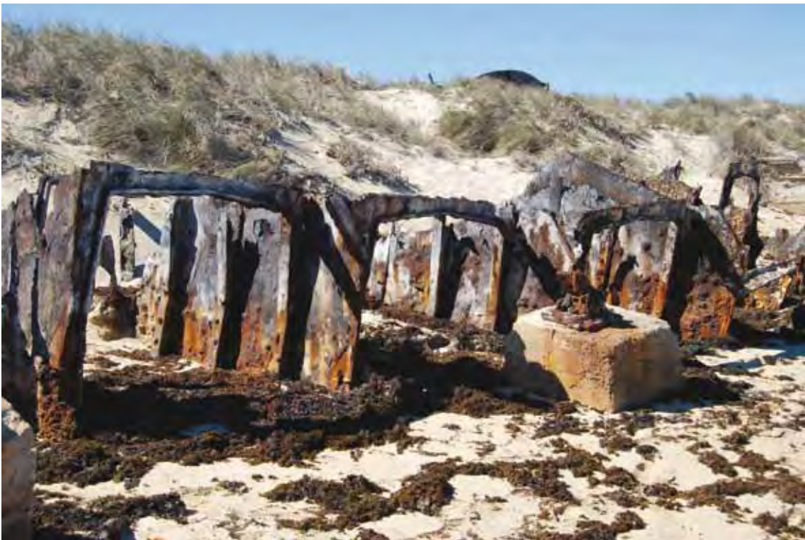
Figure 39. Rusted remains of oil receiving/storage tanks 2009 (Myra Stanbury).
