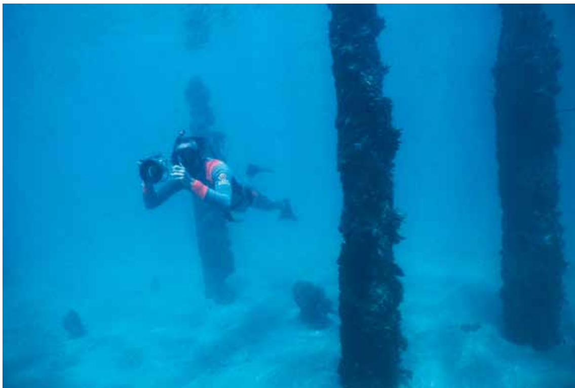
Figure 62. The jetty piles at Maud Landing (Patrick Baker).
