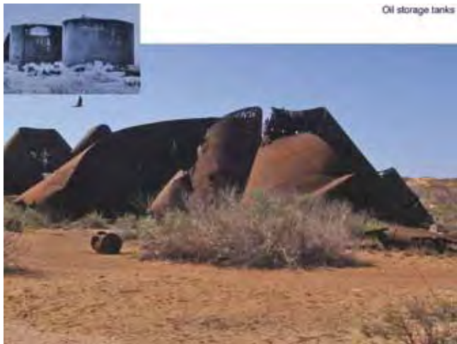
Figure 19. Oil storage tanks (Colin Cockram).
