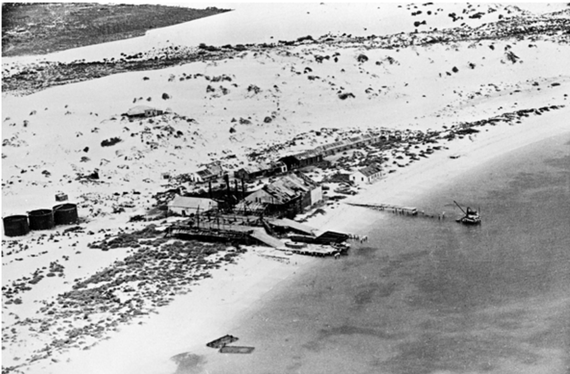
Figure 9. Aerial photograph of the Norwegian Bay Whaling Station in 1946 (from the Stanley Fowler Collection, courtesy of R.G. Chittleborough).
