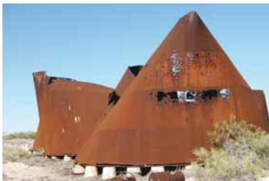
Figure 49. Oil storage tanks supported on cement barrels, viewed from the north-east (Myra Stanbury).
