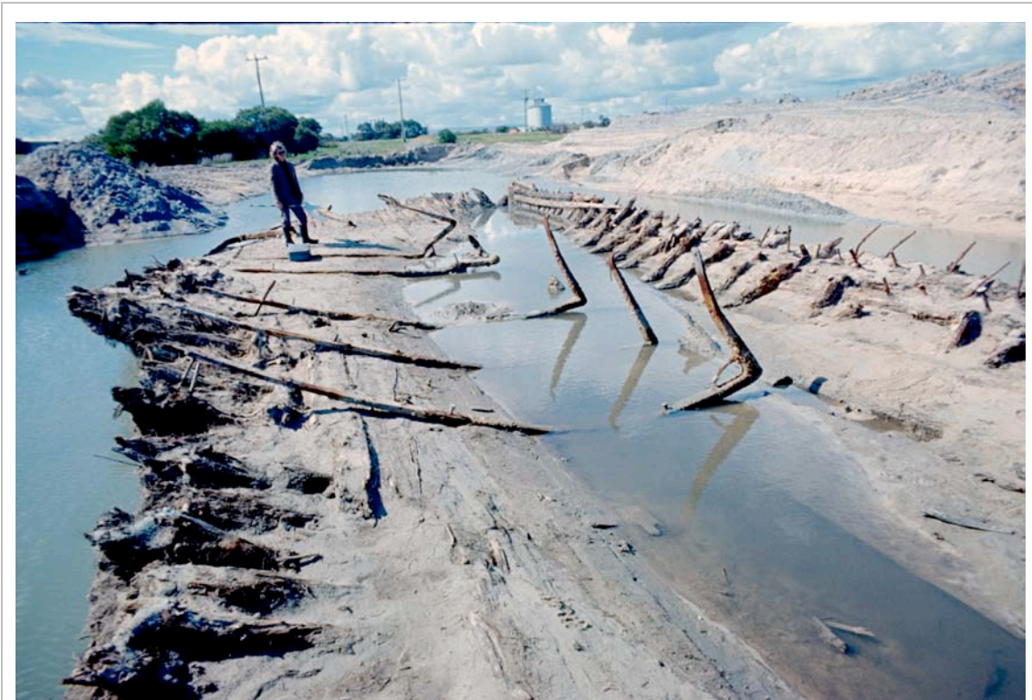
Image: Upper port hull section of Solglyt , found in 1973 before being removed. (NOTE: the iron knees)
