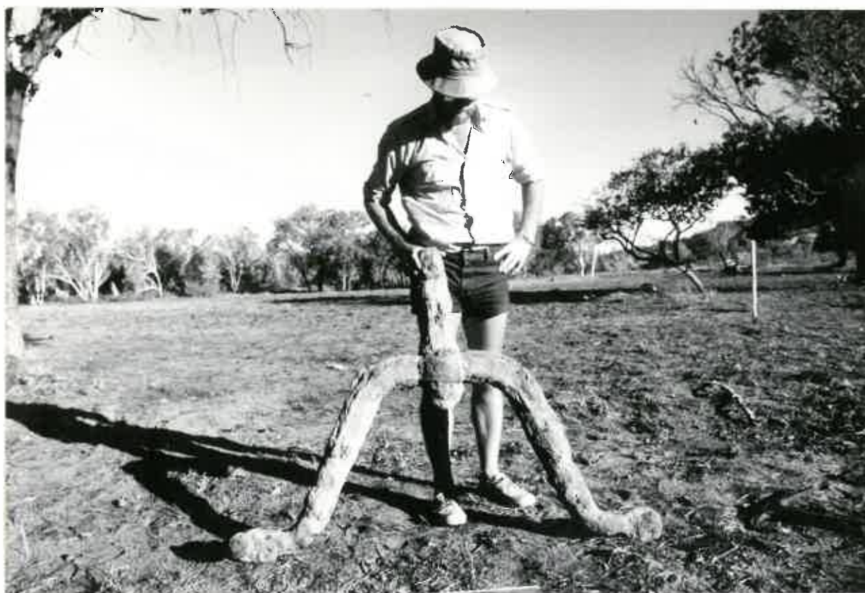
13) yard truss from Fishermans Bend.
