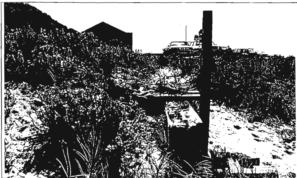
Figure 5. Land remnants of the Hopetoun Jetty looking north. (D. Cumming, April 1994.)
