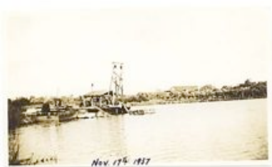
Figure 6: Photograph of two dredges together taken 17 November 1937—grab dredge at left and suction dredge at right. (City of Wanneroo Museum and Heritage Collection)
