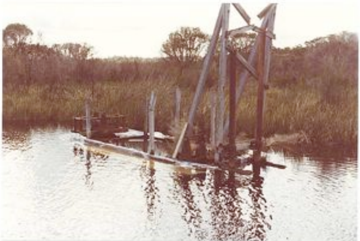
Figure 7: Photograph of northern site suction dredge dated 1983 (City of Wanneroo Museum and Heritage Collection)
