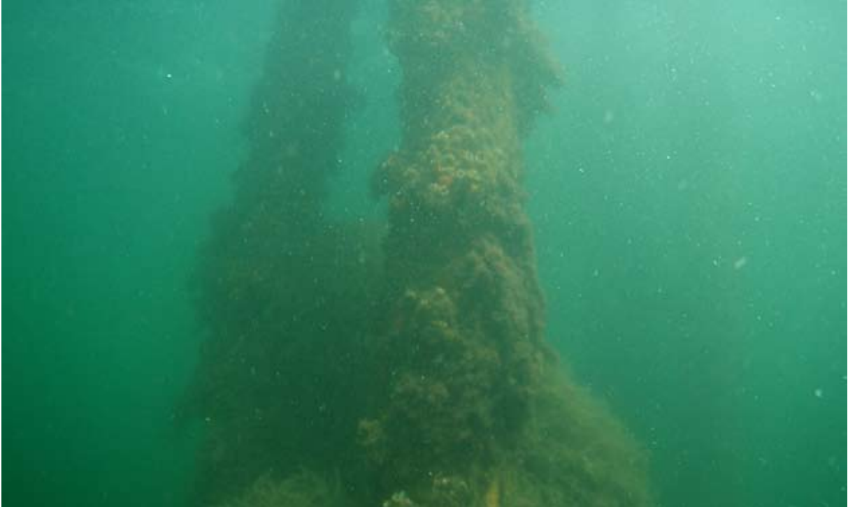
Figure 8. Modern jetty pile.
